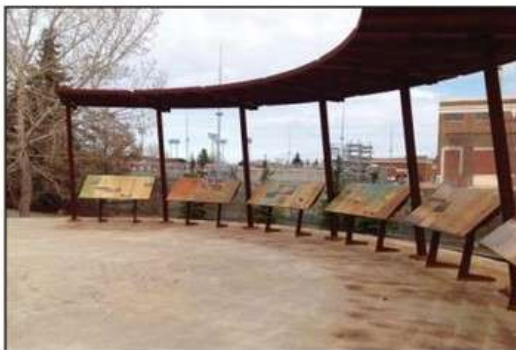
Interpretive Belvedere prior to relocation
