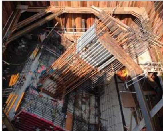
Anchor rods will support bridge arches
