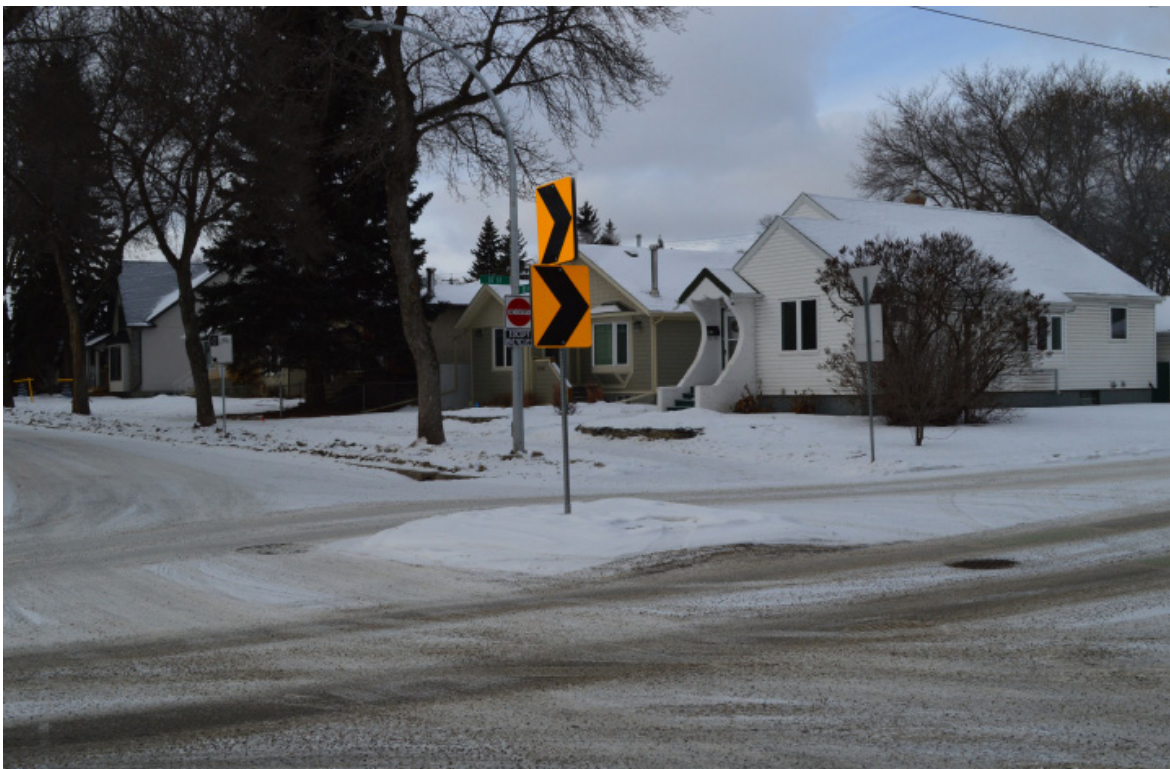
Figure 14: Traffic calming infrastructure on 83rd Avenue and 97th Street
